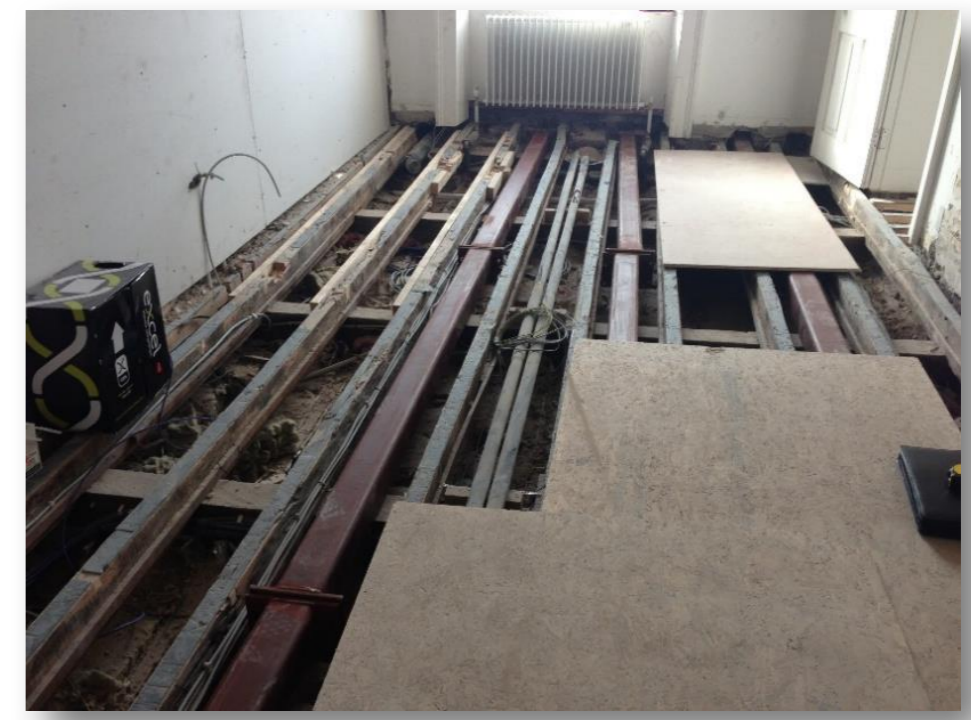
Example of In Line Strengthening
