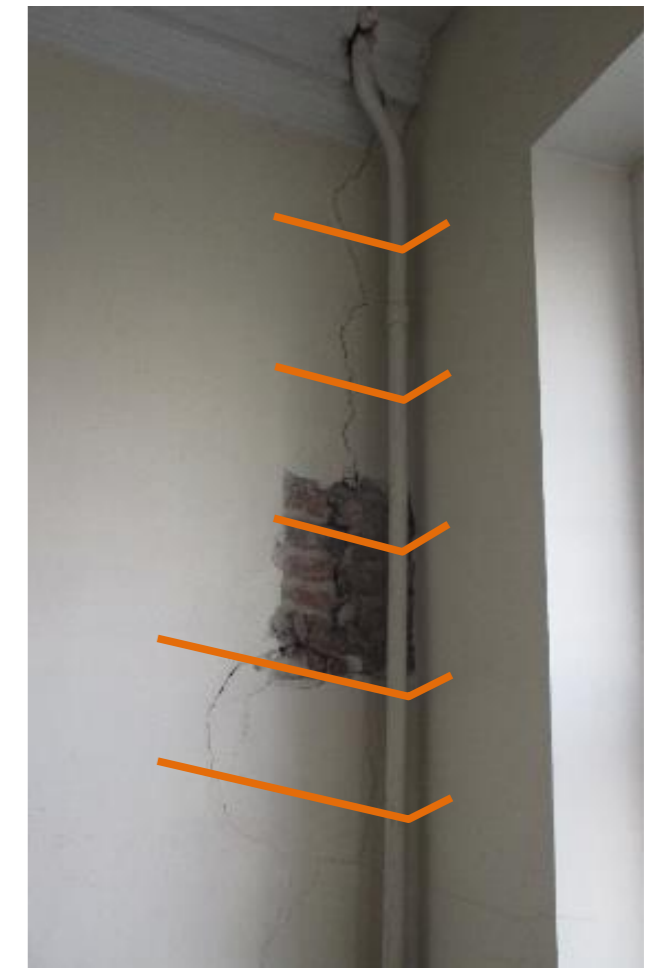
Strengthening of Walls
